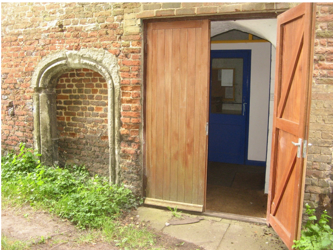
Fig 10 Gatehouse: Blocked doorway and remains of a second doorway, much altered and enlarged, alongside; floor level was originally lower
