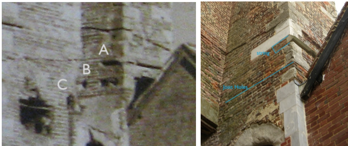
Fig 24 The north-west stair tower at second floor level in 1934 and 2017 showing (A) weathering course returning but now cut off; (B) gallery roof joist sockets now lost; (C – 1934 only) socket for bead of timber frame of west wall of the west gallery. Note extensive survival of internal plasterwork below joists 'B' in 1934; barely a fragment now remains
