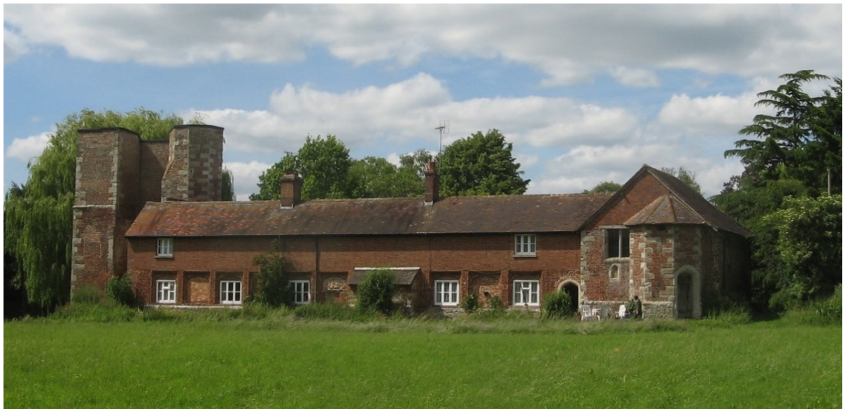
Fig 8: The north-west range of the outer court as it currently exists
