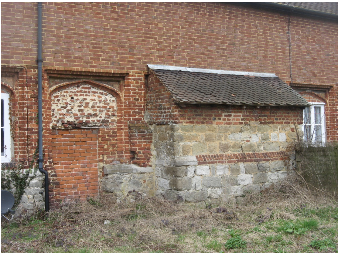
Fig 17 The projection on the south side of the north-west range; note the section of the plinth raised in brick, and the chamfered jamb of a doorway formed through one of the arched openings of the cloister. The rough infill above it is of uncertain date, the infill of the doorway around 1800
