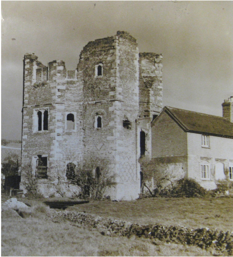
Fig 23 The north-west tower in 1934, after the removal of ivy (SPAB archive)
